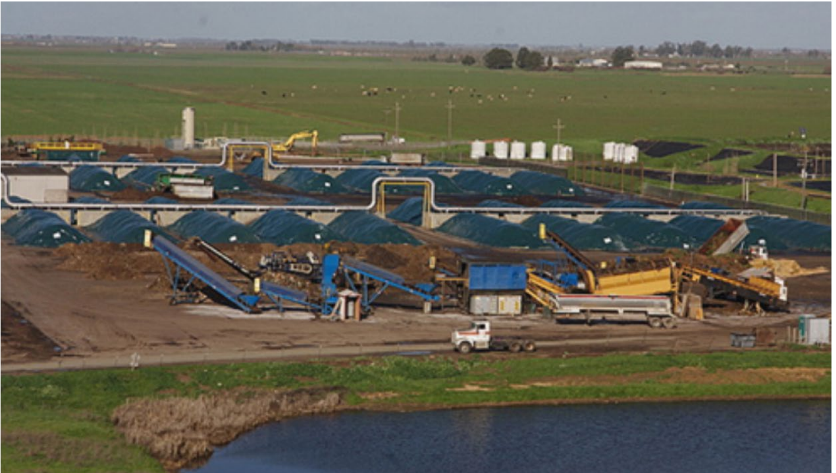
Engineered Compost System (ECS)
